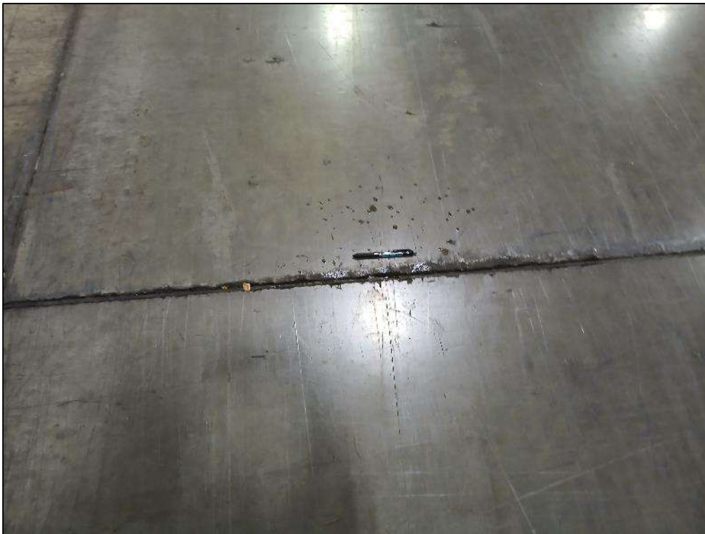
Photo 2: Photo of a gap in the caulk along a concrete seam near location A133.
